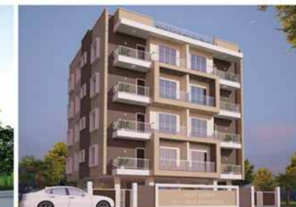
WEST AVENUES Ayyappa Nagar, Nagpur
