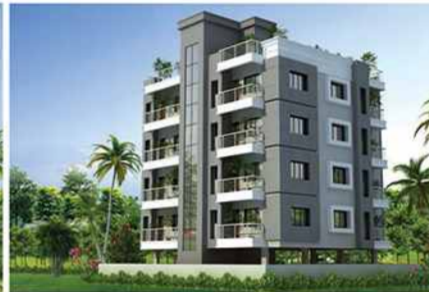
THE RADIAN Beside St. Vincent Pallotti School, Nagpur
